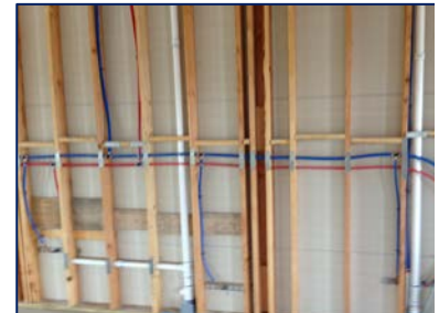
Uninsulated Wall Cavity
