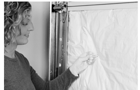
Install Retention Clips
