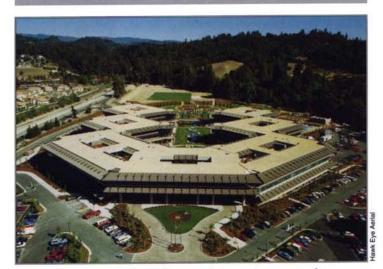
Meets or exceeds building code requirements for most types of commercial construction. The impressive Borland International Complex in California was constructed with a Sprayed Polyurethane Foam roofing assembly. The SPF assembly has fire-resistance ratings that meet or exceed most commercial building code requirements, so it can be included in new construction plans for most every type of commercial structure and type of occupancy.
