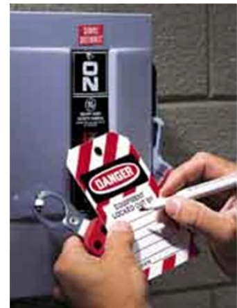
FIGURE 3 - Deactivate and mark HVAC system at electrical panel (use LOTO procedure and indicate date, time and name of person applying the tag)
