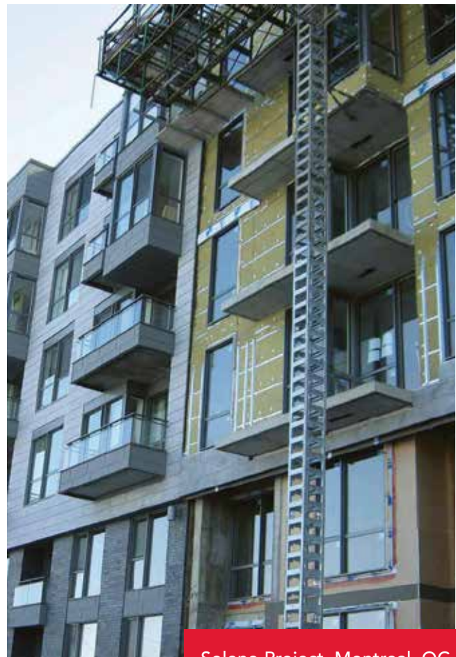
Soleno Project, Montreal, QC ROCKWOOL Cavityrock®
